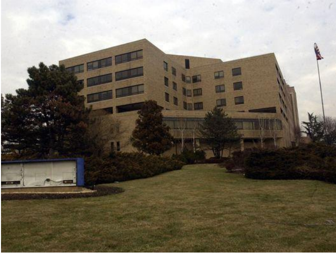
The former United Hospital in Port Chester.
